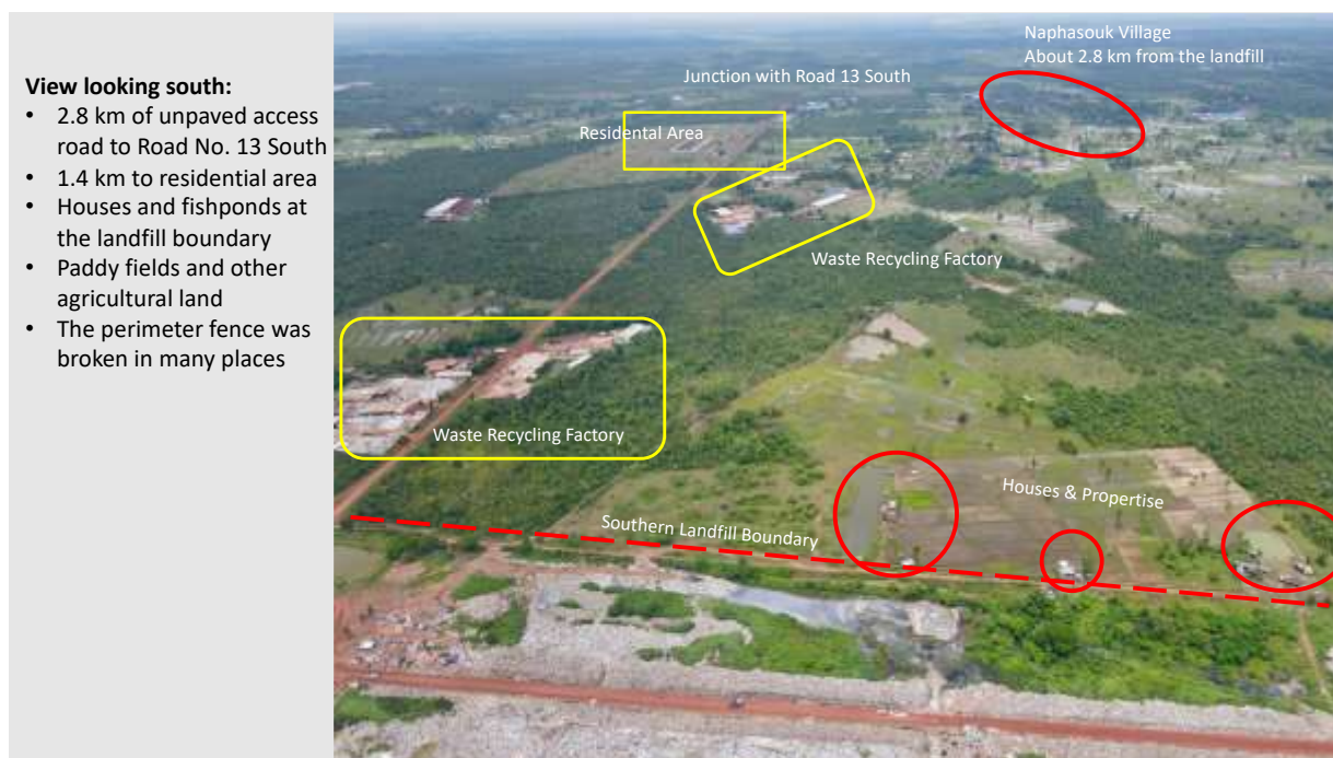
FIGURE 7-1 DRONE PHOTO WITH VIEW FROM THE LANDFILL LOOKING SOUTH (JULY 2022)
