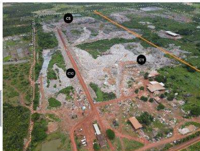
Km32 Landfill, Looking West
