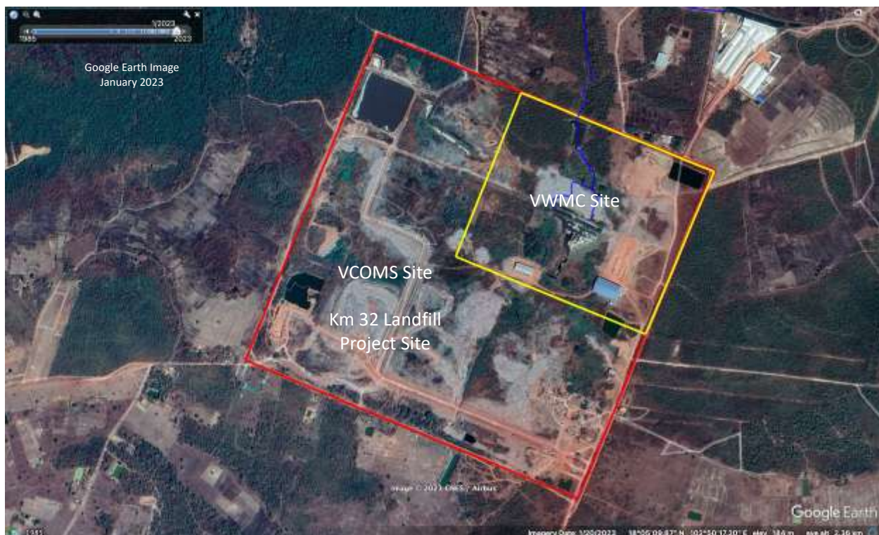
FIGURE 0-2 THE KM 32 LANDFILL SITE
