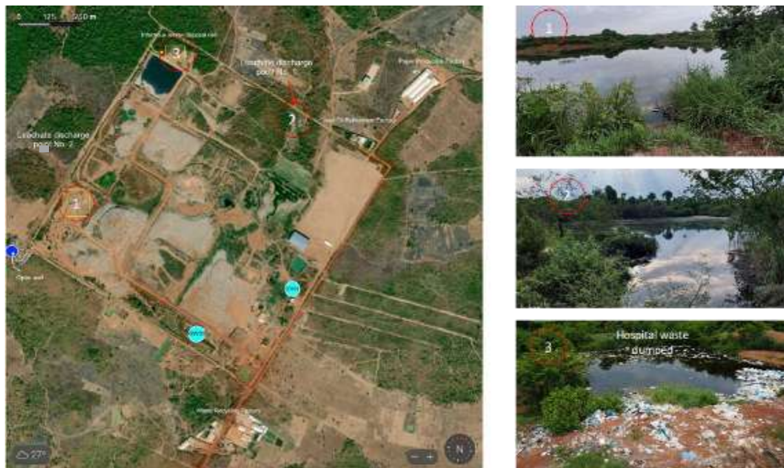
FIGURE 0-6 LEACHATE DRAINAGE FROM THE KM 32 LANDFILL
