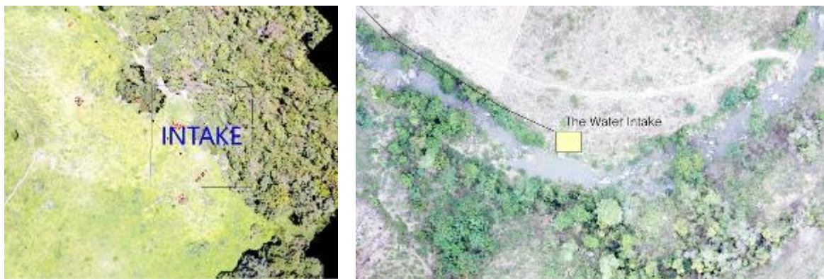
Figure 3-6 Aerial Picture of Water Intake of Namthae WSS(a) and Phieinghong WSS (b)
