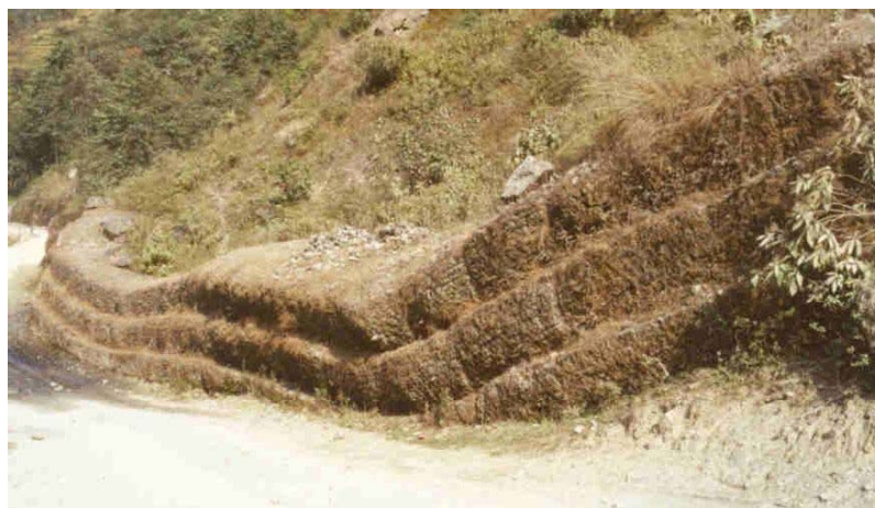
Figure 5-13: Gabion retaining wall – still functioning despite major slope movements
