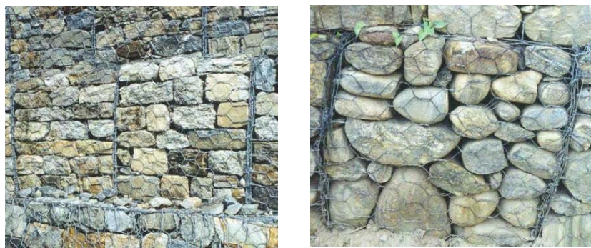
Figure 6-5: Examples of good and poor stone filling
