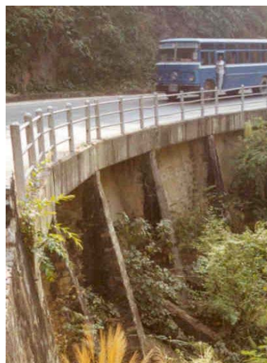
Buttressed masonry wall with reinforced concrete road slab
