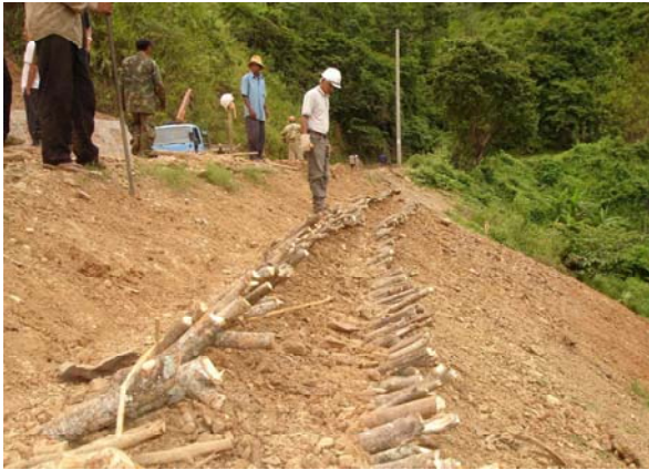
Figure 6-9: A freshly completed section of single-row brush layer
