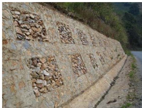
Figure 5-5: Typical composite masonry wall
