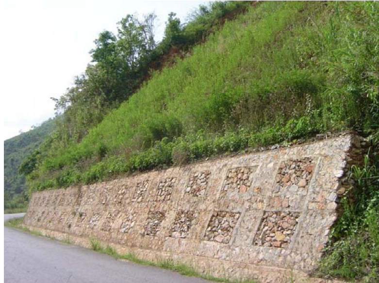
Figure 4-18: Typical bio-engineering measures to prevent surface erosion
