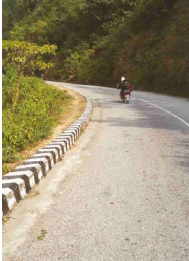
Figure 4-12: Kerb to road edge
