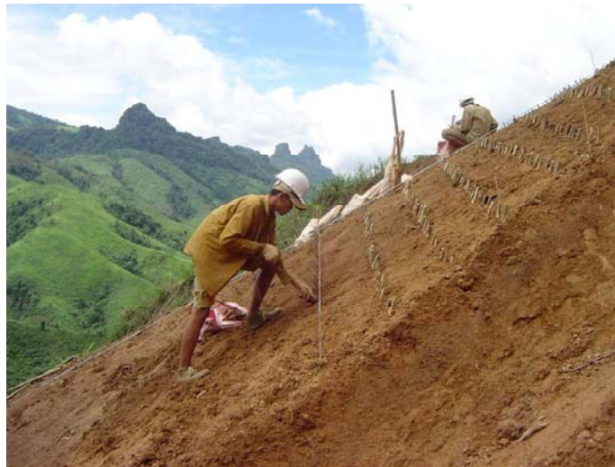
Figure 6-8: Planting lines of grass on a trimmed landslide head scarp
