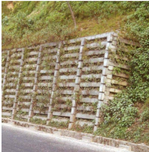
Concrete Crib Wall
