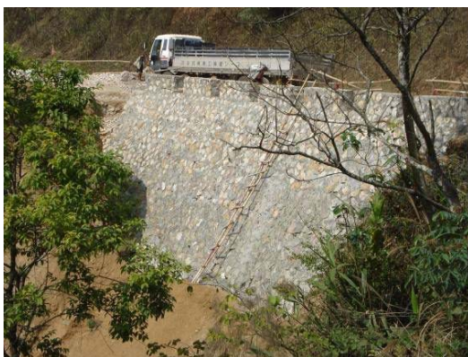
Figure 5-7: Typical mortared masonry wall
