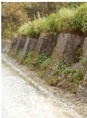
Buttressed mortared masonry wall
