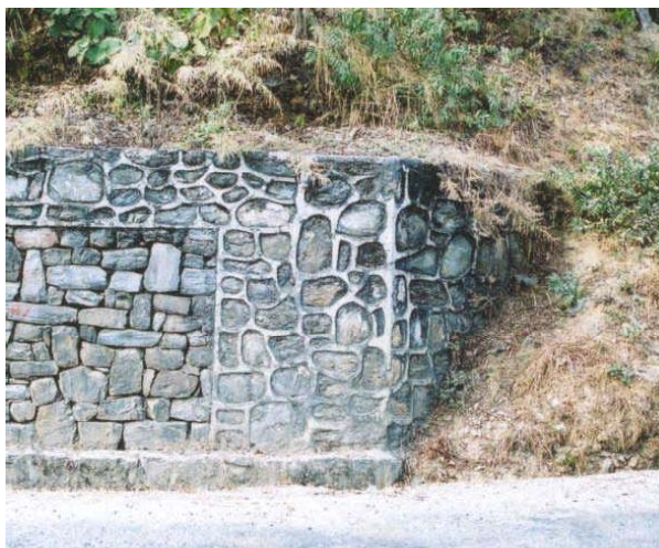
Figure 6.3: Retaining wall with angled return
