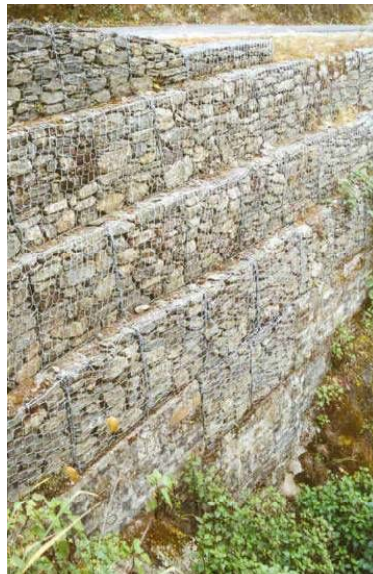
Figure 5-14: Gabion wall on stepped masonry base
