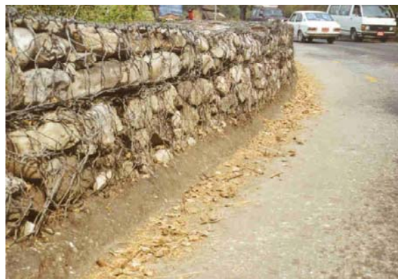
Figure 5-11: Bituminous upstand to gabion road supporting wall
