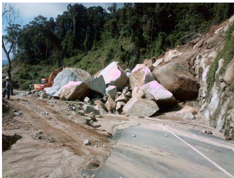
Figure 2-8: Rockfall on Road 18b
