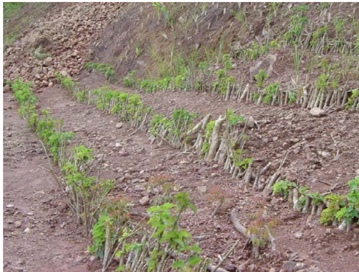
Figure 6-11: A palisade about 2 months after planting
