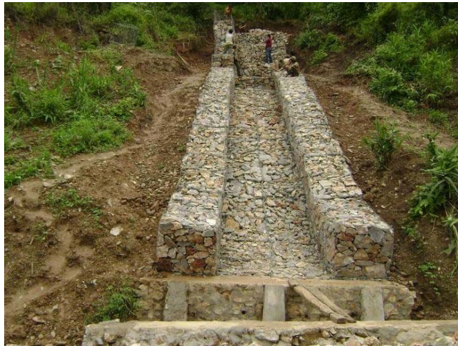
Figure 4-16. Typical gabion chute
