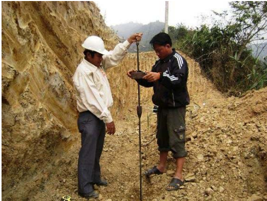
Figure 3-6: Dynamic Cone Penetrometer test
