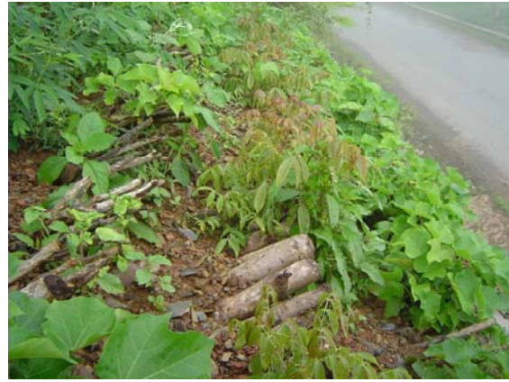
Figure 6-10: A brush layer about 3 months after planting
