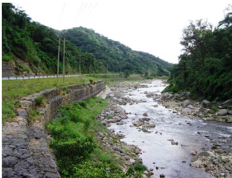
Figure 4-17. Typical gabion river training works
