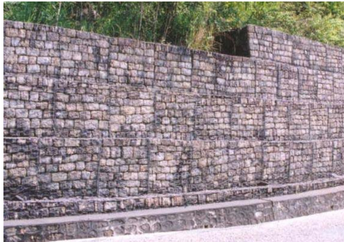
Figure 5-10: Typical gabion wall
