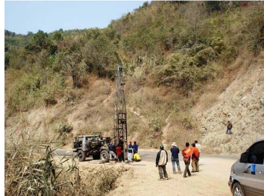
Figure 3-7: Site investigation using drill rigs
