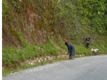
Clearing drains
