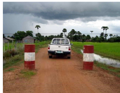
Concrete side posts
